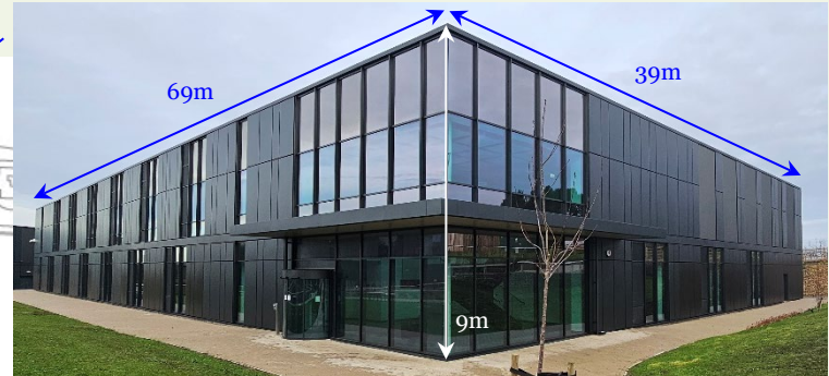
New Filtronic footprint adding ~90,000 sq ft over three floors, operational from early 2026
