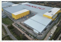
Tsukuba Robot Factory #1/Finished products warehouse
